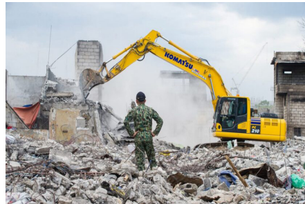
A backhoe demolishes the remaining structures in the fire-gutted community in Brgy. Pinyahan, Quezon City.
